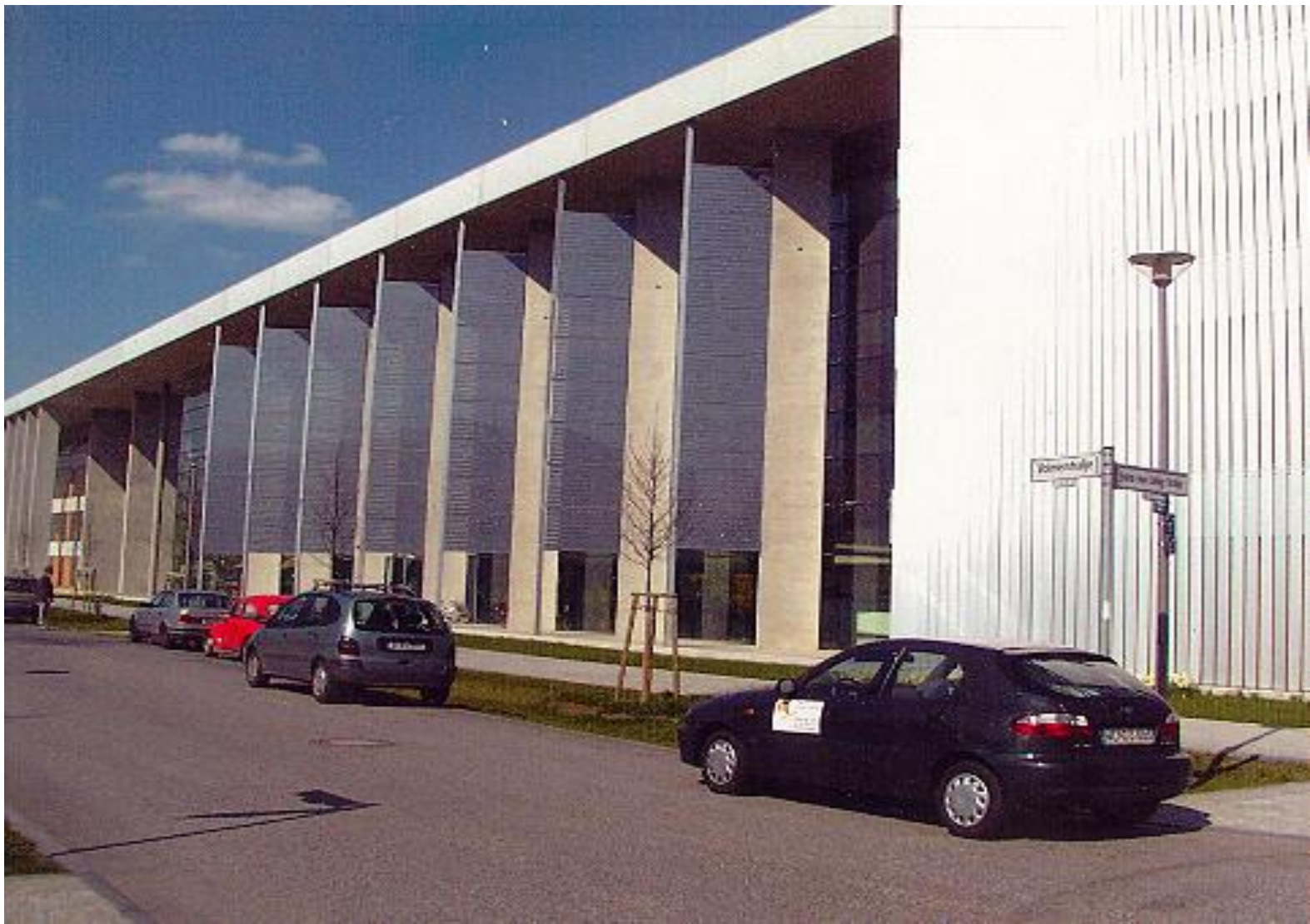
PV-Facade of the Center for Environmental-, Bio-, and Energy Technology, 14 kW p , 1998, AstroPower Si-Apex-cells, Modules made by SOLON
