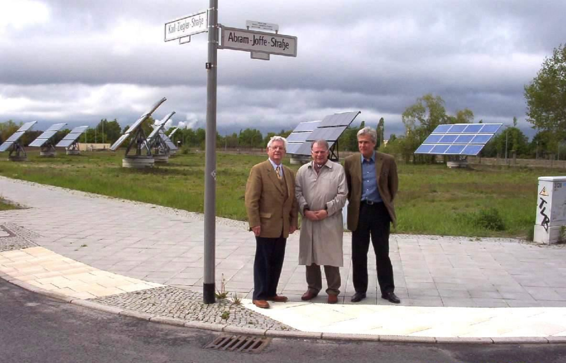
10 Solon Movers at Abram Ioffe Street, Each approx. 7 kW p , Installed in 2004 From right: Hardy Rudolf Schmitz, Zhores Alferov, Klaus Thiessen
