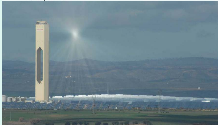
Solar Power Tower Example: PS 10
